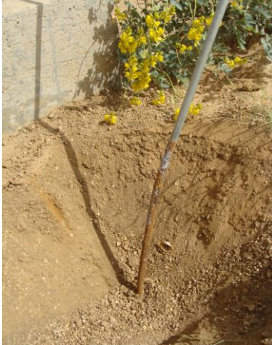
Figure 8. Part of round zinc galvanized steel earth conductor after 6 months service (partially embedded in soil).
