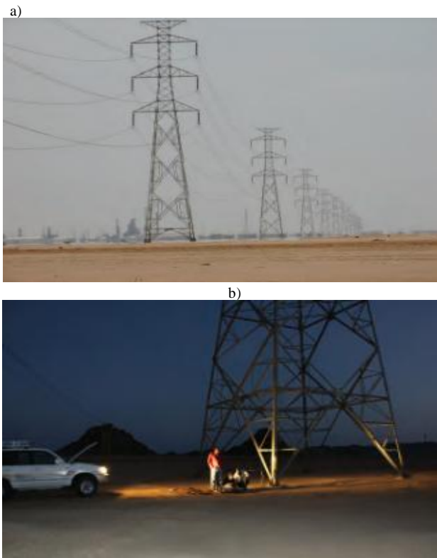
Figure 2. General view (a) and tower nr 31 (b) at investigated site.
